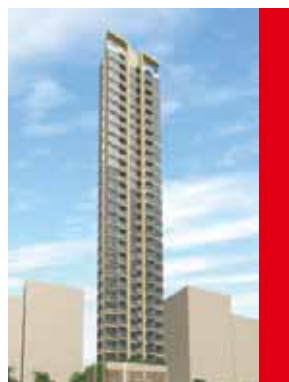
No. 287-293 Sai Yeung Choi Street North Sham Shui Po, Hong Kong
