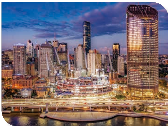
Construction at Queen's Wharf, Brisbane
