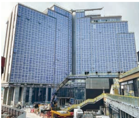
Construction at Dorsett Kai Tak, Hong Kong
