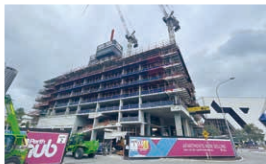
Construction at Perth City Link
