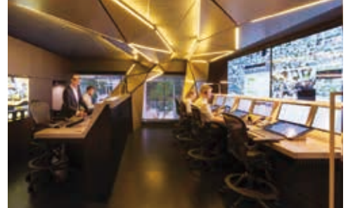
Central monitoring system, Care Assist
