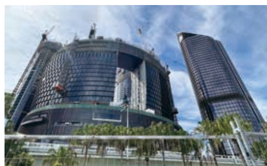
Construction at Queen's Wharf Brisbane
