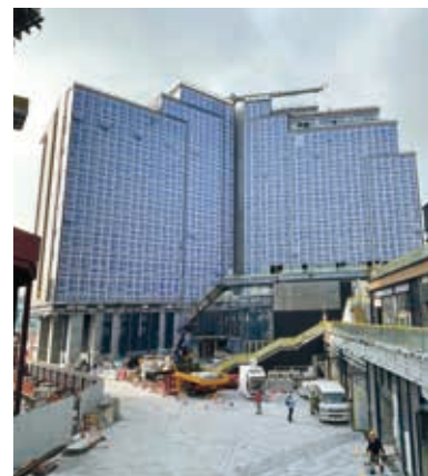
Construction at Dorsett Kai Tak, Hong Kong
