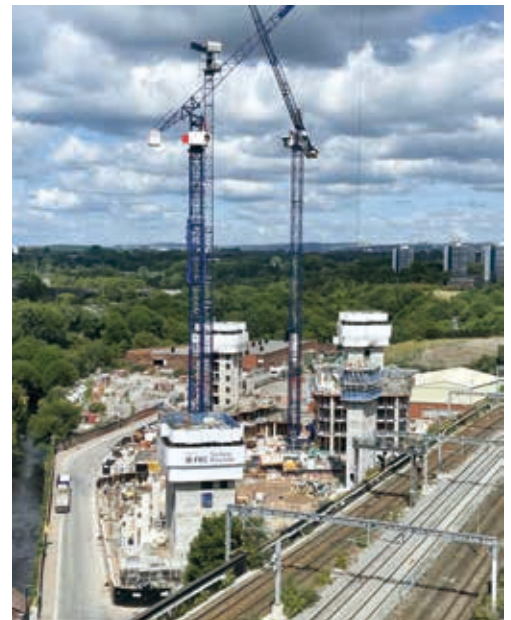
Construction at Victoria Riverside, Manchester
