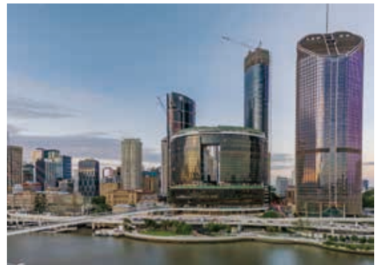
Construction at Queen's Wharf Brisbane, Brisbane
