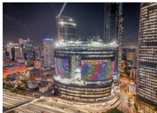
Construction at Queen's Wharf Brisbane, Brisbane
