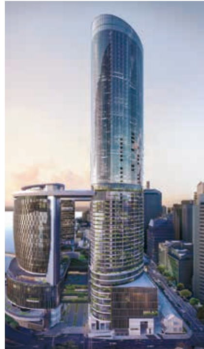
Queen's Wharf Residences – Tower 4, Brisbane
