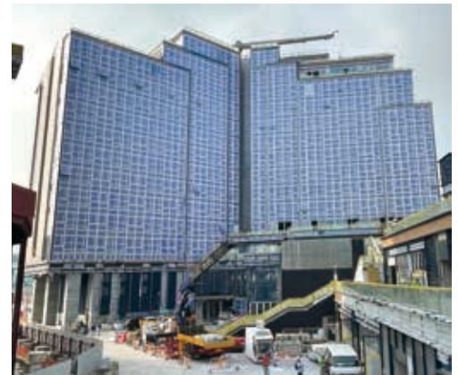
Construction at Dorsett Kai Tak, Hong Kong
